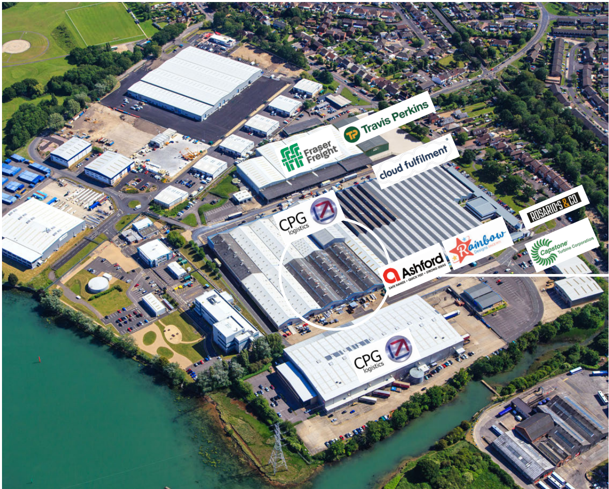
Aerial photograph of Fareham Reach Business Park looking south west.
