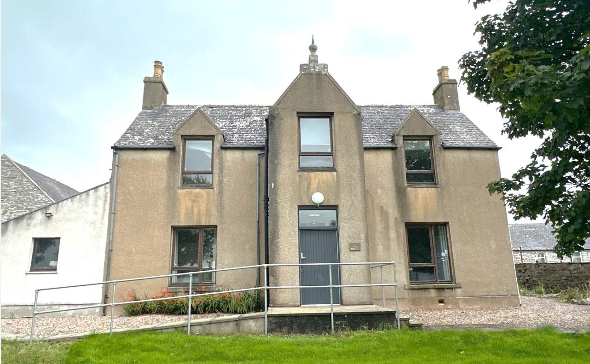
FORMER SCHOOLHOUSE, MAIN STREET, LYBSTER
