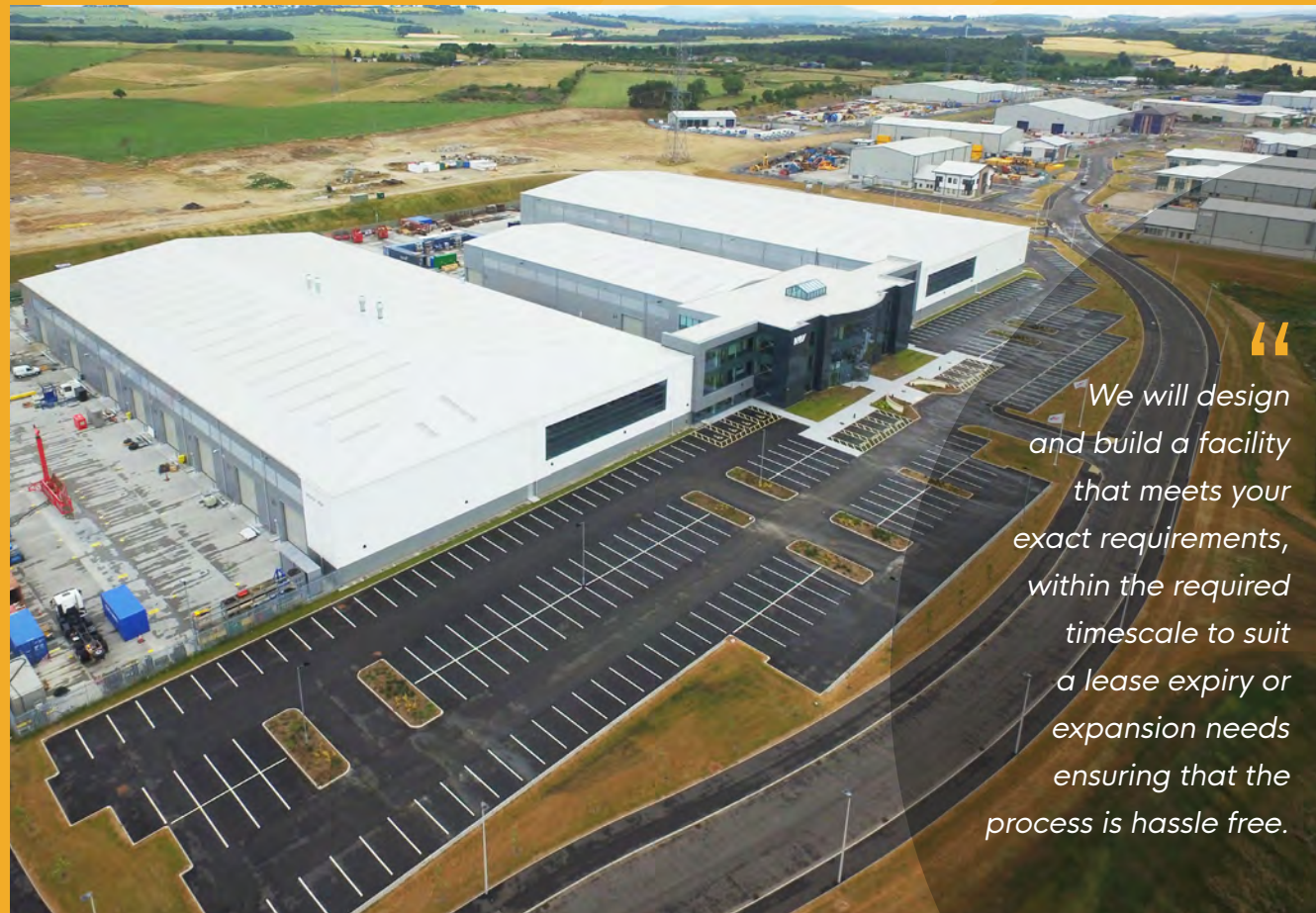
NOV FACILITY AT MIDMILL BUSINESS PARK, COMPLETED 2018 BY MALCOLM ALLAN.
