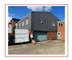
elevations to ground floor and profile steel clad to first floor and roof. The first floor is of concrete plank construction with adequate floor loading for light industrial use. The current occupiers have fitted out half the first floor as offices, but these could easily be removed, or extended. Externally, there are 5 car parking spaces and an electrically operated access door. The property provides highly flexible accommodation suitable for a variety of industrial and / or office uses.
