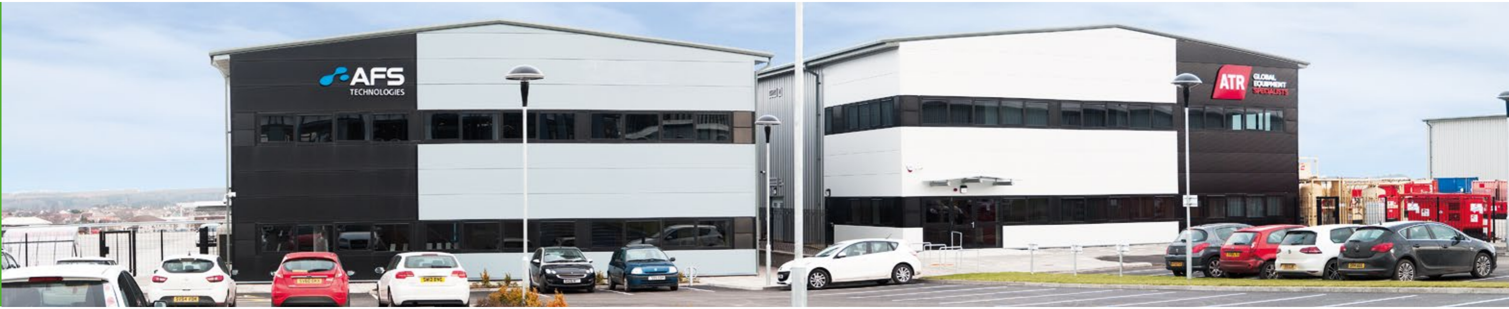
OFFICE AND WAREHOUSE 3 & 5 INTERNATIONAL AVENUE
