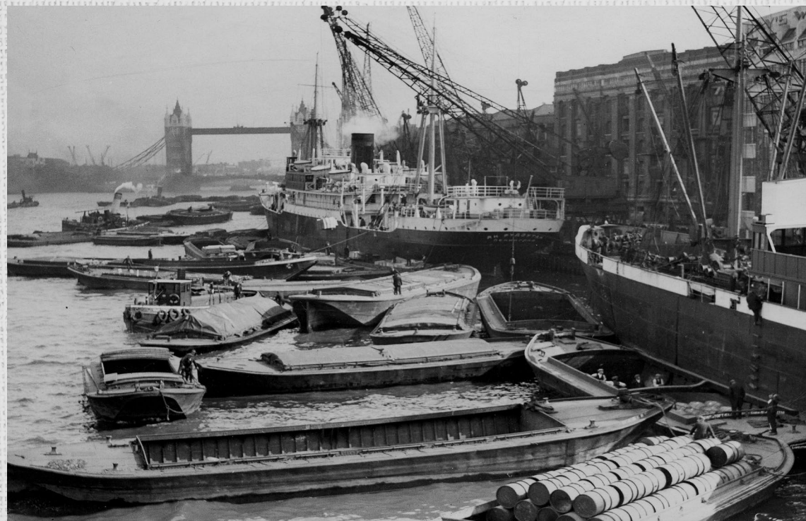
1935 Barges moored at Hay's Wharf.
