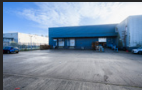
Rear Dock and Level Access Loading Doors
