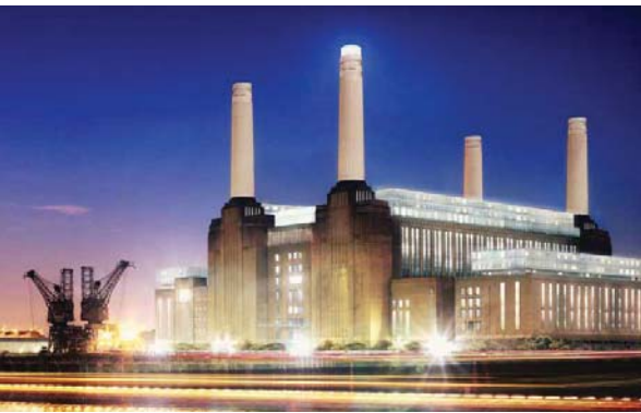
EXTERNAL VIEW OF THE CHIMNEY LIFT
