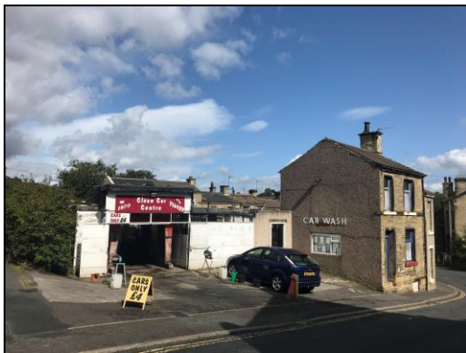
Valeting Centre & Office
