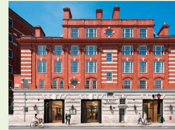
WESTMINSTER FIRE STATION SW1
