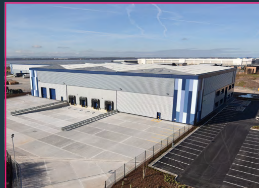
HURRICANE 52 Estuary Business Park, Liverpool
