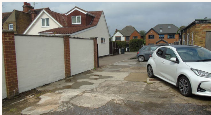
SERVICE ACCESS/REAR YARD
