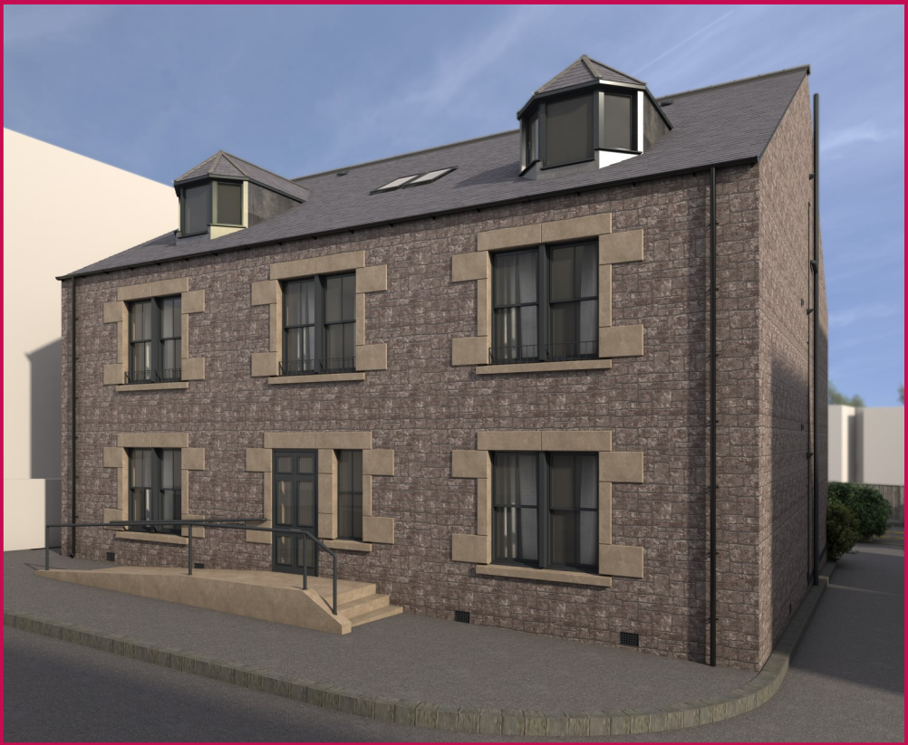
Front View (from Millar Street)
