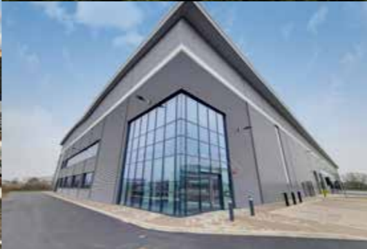
ASCENT LOGISTICS PARK LEIGHTON BUZZARD Eight warehouse / industrial units 14,140 to 123,490 sq ft - FULLY LET
