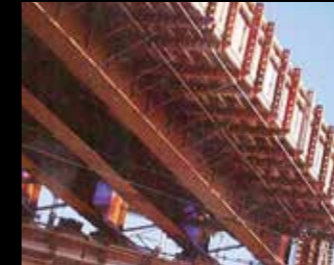
FARRRS bridge beams spanning the East Coast Mainline
