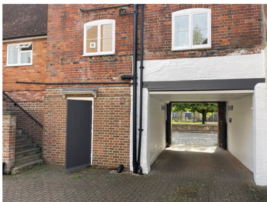
Rear Entrance / Storage
