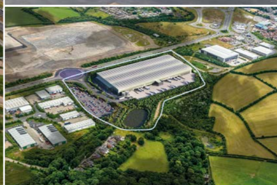
Barnsley 340 340,000 sq ft Grade-A logistics unit
