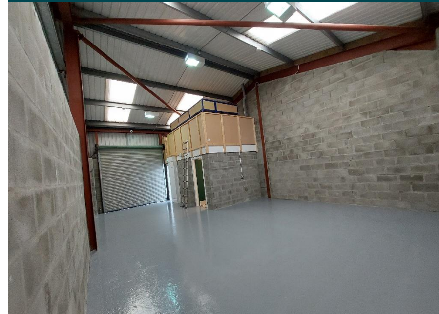
Warehouse (indicative post refurbishment)
