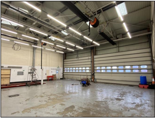
Fleet Garage, Cheney Manor Road, Swindon, SN2 2QB
