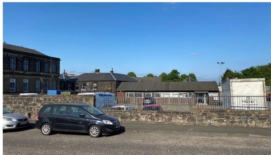
Outdoor Education Building from West
