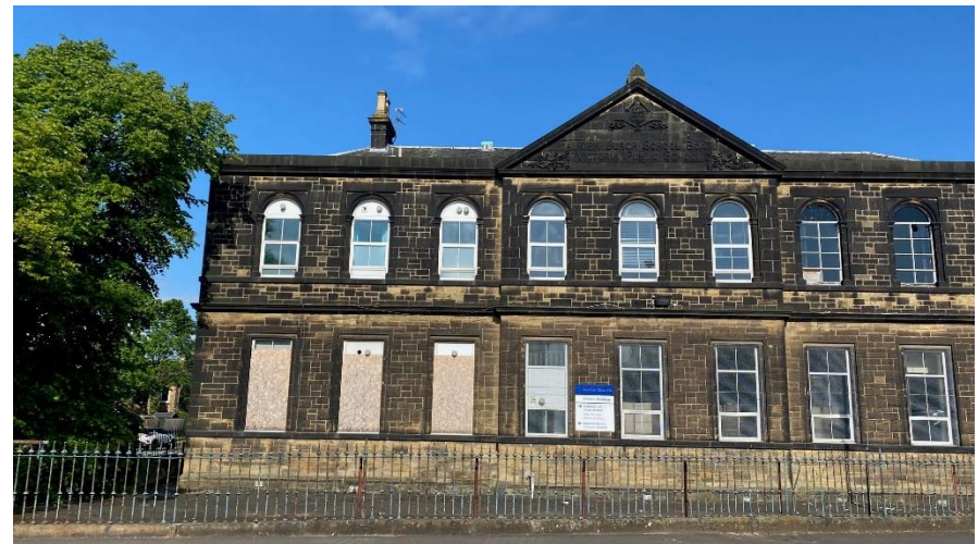
VICTORIA BUILDINGS FROM WEST
